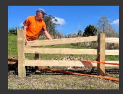
Tap on the new post to the rails using the rubber mallet or small sledge hammer (use a piece of scrap timber between the post and small sledge hammer to avoid damaging the post), **ensuring**
