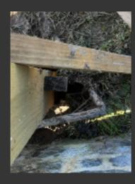
In the pictures above Tom has used stakes both ways as well as a couple of timber off cuts in the hole either side to help eliminate any lateral movement or the post turning in the hole. In this case Tom had a stone wall to put some timber between the post and the stone wall, if you don't have anything like this, another stake could be used.
