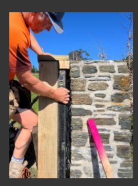
Secure this post once you have it level for the two vertical planes, either by ramming the earth back **2.4** - around the post or securing with stakes if using concrete to secure your posts. It is important to secure this post very well to help eliminate movement when tapping in the rails for each section.
